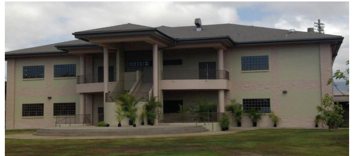
Saber Hall, a new 8-classroom building at James Campbell High, opens this fall.
